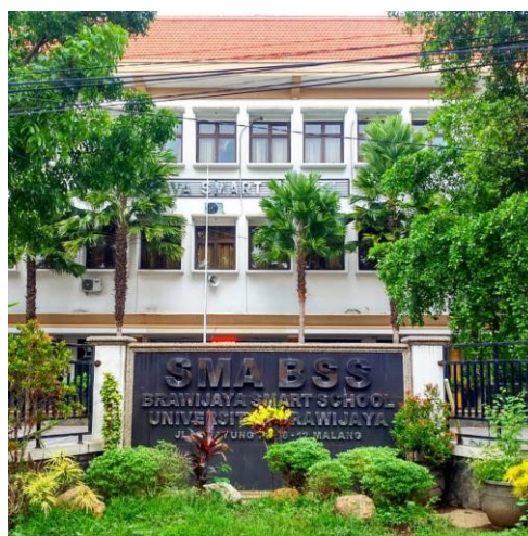
Gambar 1. SMA Brawijaya Smart School ( https://brawijaya-smart-school.business.site/ )
